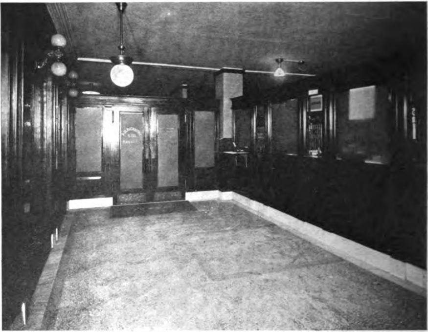
Entrance from Elevators.
